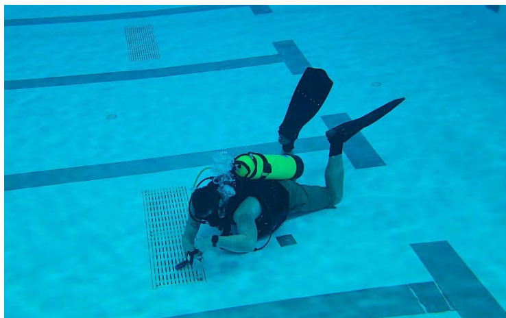
Changing Grates November 24
